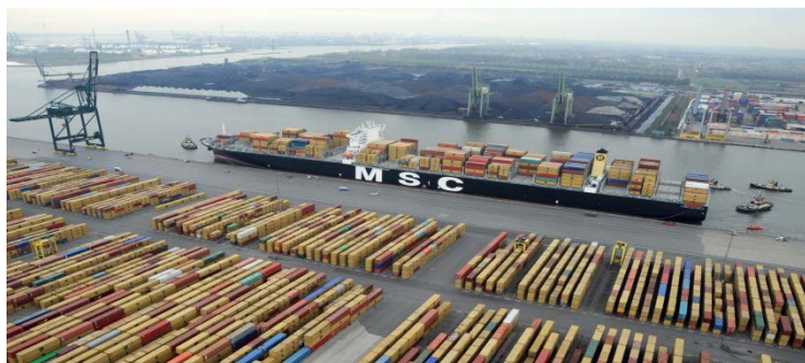
MSC Home Terminal in Antwerp, Belgium
